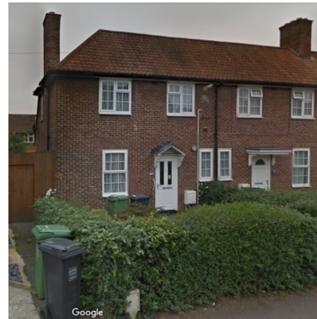
133 Cavity Wall Insulation properties across Bellingham, Downham and Whitefoot
