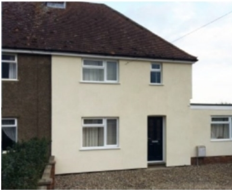
20 External Wall Insulation properties in Grove Park
